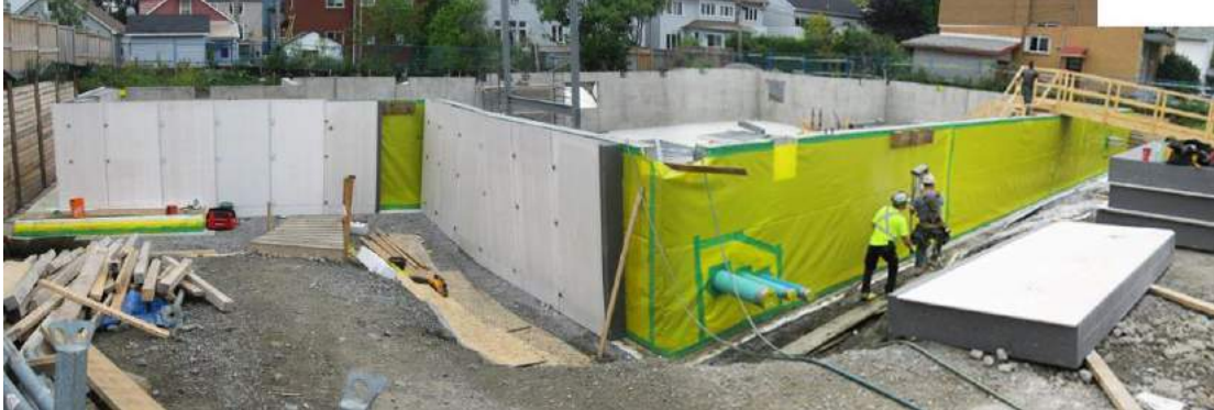
Foundation walls – Below Grade SIPs
