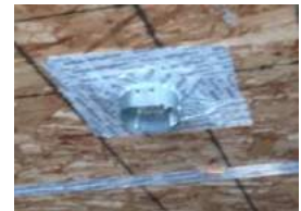
air tight installation at the Steel brackets with Siga Nail Seal Tape
