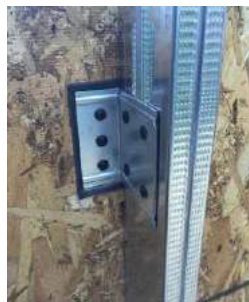
SIP Connection to St Studs
