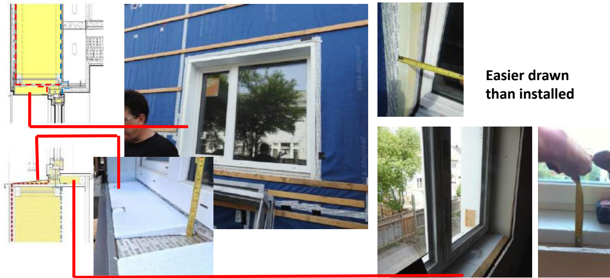
PH Windows Installation: Auxiliary Insulation
