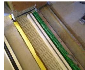
Thermo-profile underneath doors
