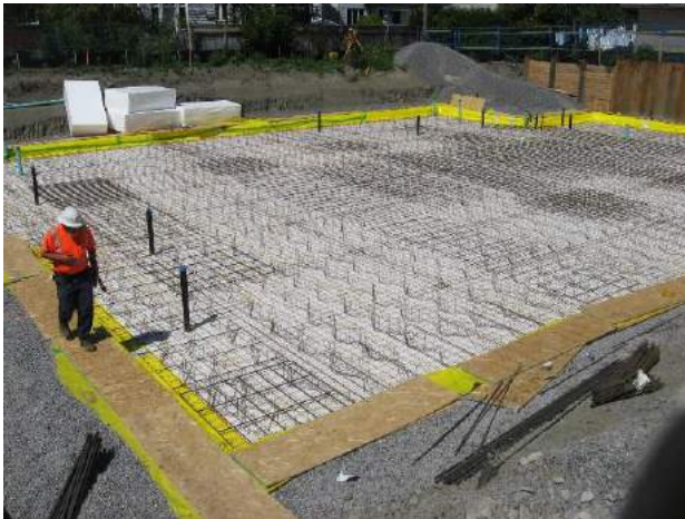
Foundations: Tray slab foundation and concrete foundation wall
